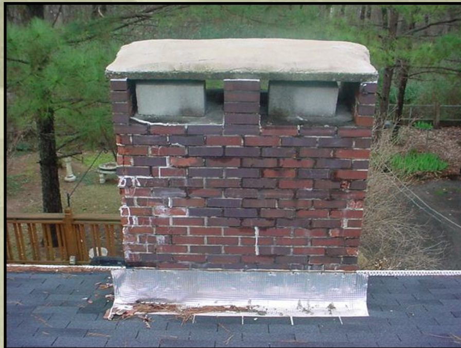
cement chimney pan
