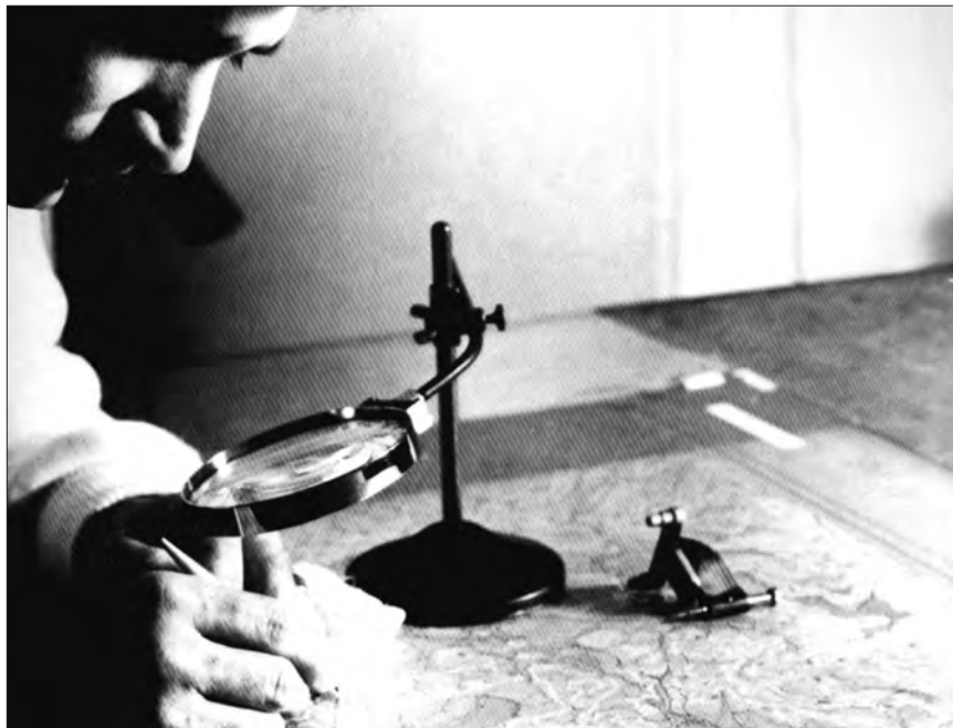
Figure 14. Scribing contour lines for topographic map by following photomechanical guide image on scribecoat with pen tool; rigid graver rests nearby on its side (USGS 1978, p. 67).
